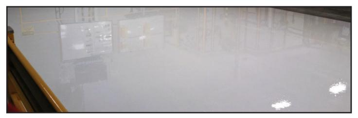
Our Water Based Urethane Gloss is a two-component (4:1) product with excellent gloss properties as well as tenacious adhesion to concrete surfaces. This product can be used as a low odor, durable solution for interior floors and surfaces. It's can also be pigmented!
