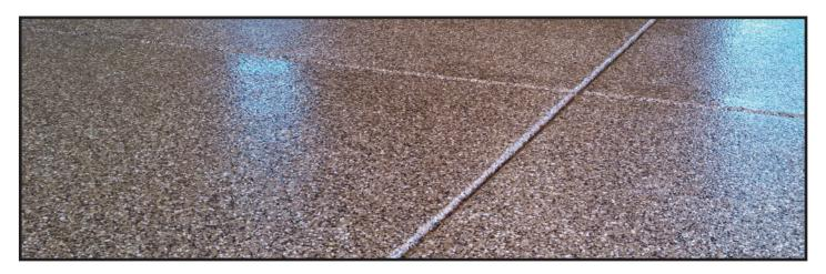
Polishing Guard is a single component, water based, high gloss protective coating specifically for use in the grinding and polishing of concrete. This product can also be put on as a standalone protectant on interior concrete floors This product utilizes both a copolymer sealer and lithium silicate densifier technology to offer concrete a UV stable, breathable protection that will not peel, flake, or yellow. This is a low VOC product.
