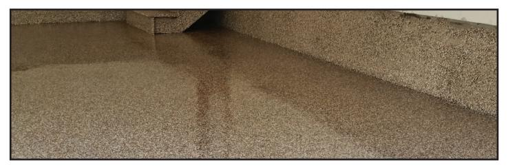
Poly base 98 is a low odor, 98% solids, two-component polyurea designed as a base-coat/primer for high-performance coating systems. Poly base 98 has an extended open time which allows users to coat larger areas prior to broadcasting chips or quartz.
