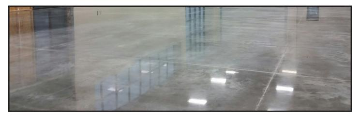
Polishing Guard is a single component, concentrated, water based, high gloss protective coating specifically for use in the grinding and polishing of concrete. This product can also be put on as a standalone protectant on interior concrete floors This product utilizes both a copolymer sealer and lithium silicate densifier technology to offer concrete a UV stable, breathable protection that will not peel, flake, or yellow. This is a low VOC product.
